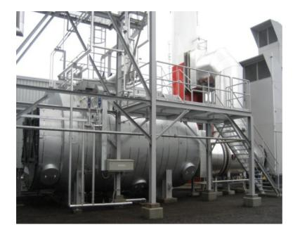
Heat Recovery Steam Generator HRSG Heat Recovery Thermal Oil Heater after Gas Generators Heat Recovery Hot Water Boiler after Gas Generators Heat Recovery Steam Generator with our partner Eck Rohr Kessel, Germany
